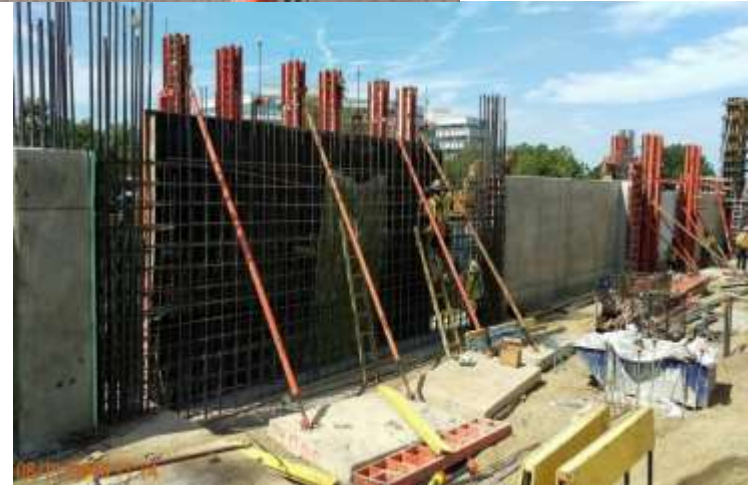
Station Foundation Walls
