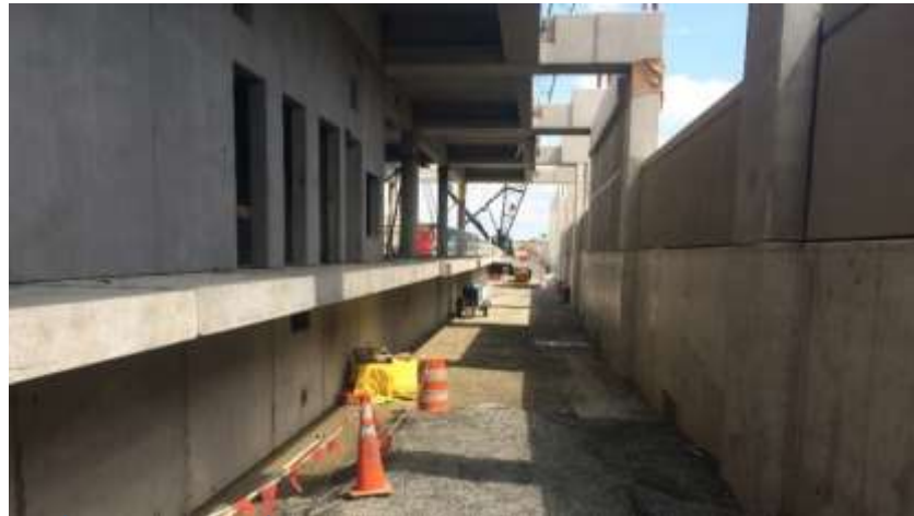
Unfinished platform and interior station wall
