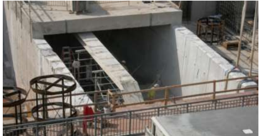
Pedestrian Tunnel to Terminal
