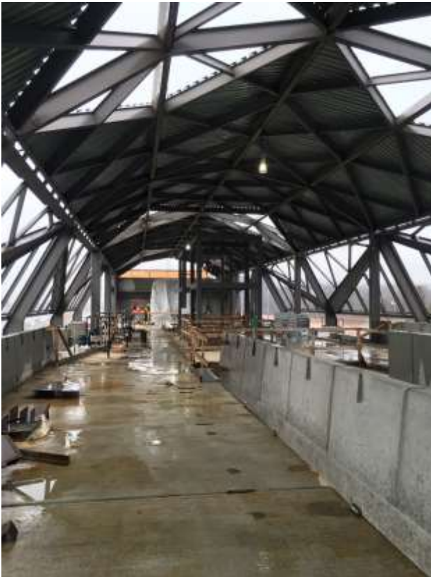
Station Mezzanine Interior
