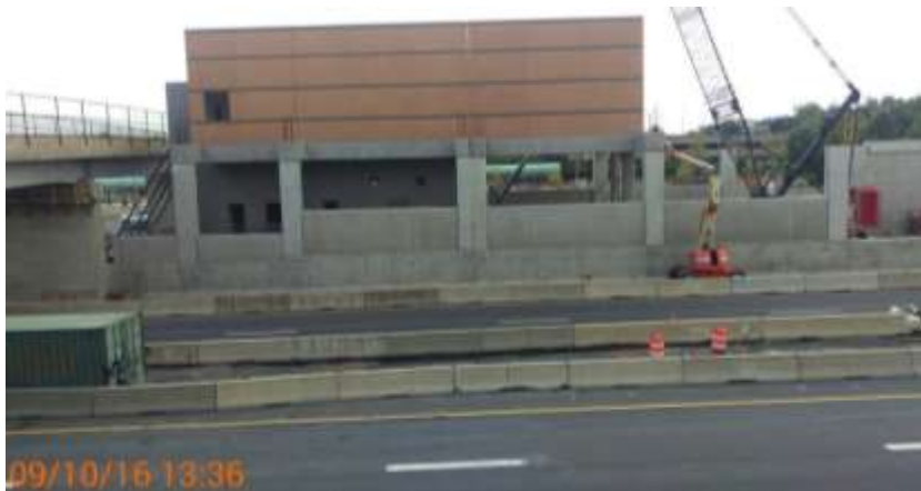
Station Barrier Walls and Exterior
